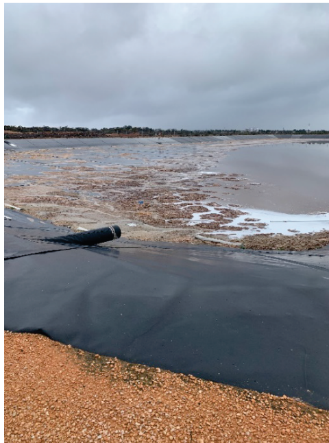
Wastewater treatment lagoon
